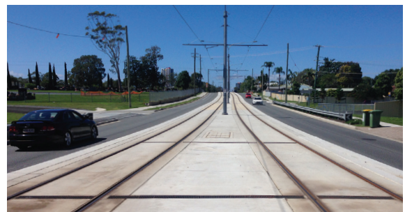
Gold Coast QLD Light Rail Project.
