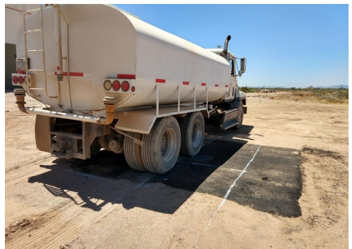
Figure 4. Loaded truck with the center of the passenger side rear tandem axle positioned where the white lines met on the asphalt pad, with a small offset.
