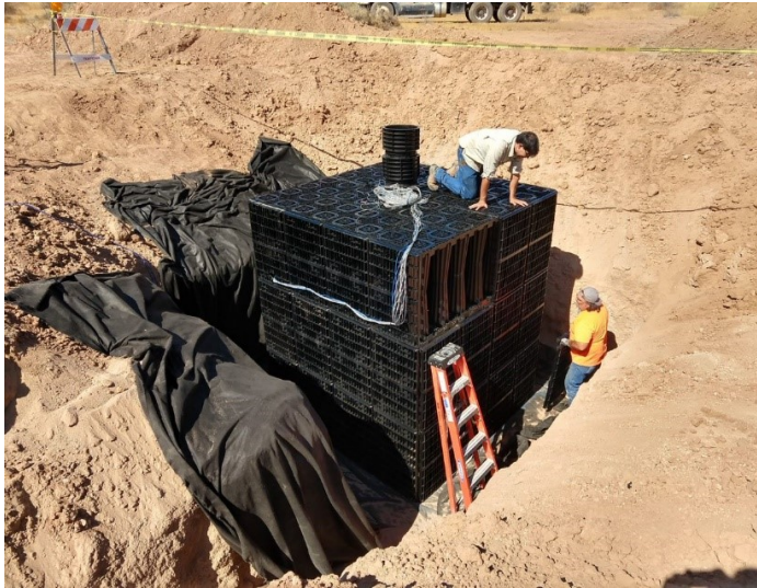
Figure 2. Three layer StormBrixx SD test structure assembled.
