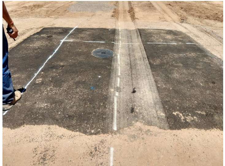
Figure 9. Rutting observed on wheel path of the asphalt surface during load testing.
