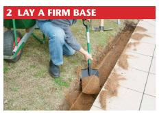
If drain is to be trafficked by vehicles, lay a bed of good quality concrete. Otherwise, use compacted fill along base of the trench.
