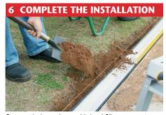
Surround channel run with backfill or concrete. Ensure that it is finished 2-3mm above grate. Remove all grates. Remove masking tape and any debris from channels. Ensure outlets are clear. Replace grates.
