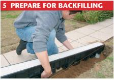
Mask along the grates over entire run length. Lower channel assembly into excvated trench, seal to drain pipe and pack to correct level.
