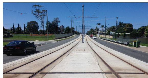
Gold Coast QLD Light Rail Project.
