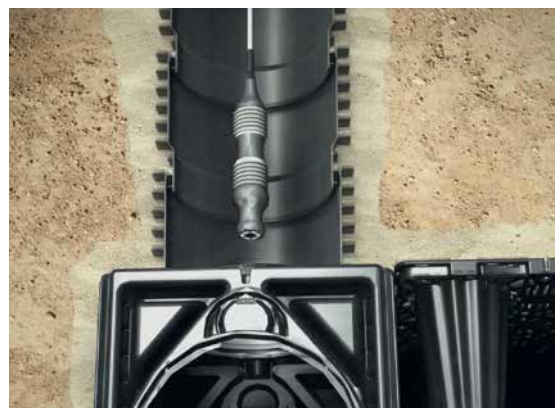
Inspection cameras are introduced into the system through the access shaft
