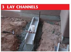
Lay channels starting at outlet. Set a string line at required height to ensure level. Seal joints if required.
