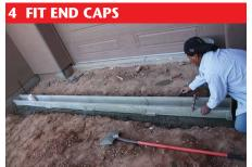
Continue to lay channels to required run length; continuously check alignment and level. Fit end caps.
