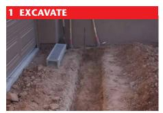
Excavate area to allow room for channels/catch basin and 100mm of concrete on all 3 sides.
