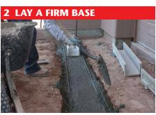
Pour concrete bed - 350mm wide by 100mm deep, keep outlet pipe clean.
