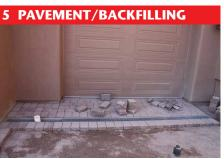
Install pavers or finish pavement surround to required level, should be 3mm above grate.
