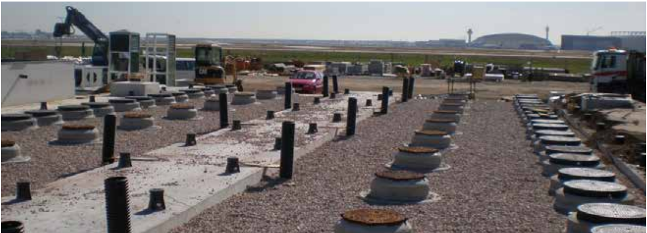
ACO light liquid separators Oleopator PR NS 100
