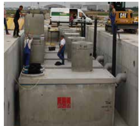
ACO light liquid separators Oleopator PR NS 100
