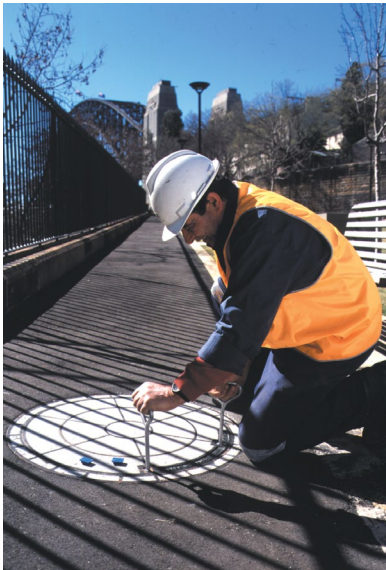
Decorative edge can be attached to the cover and frame for aesthetic areas and adds 12 or 40mm to overall height to allow for use of tiles or pavers
