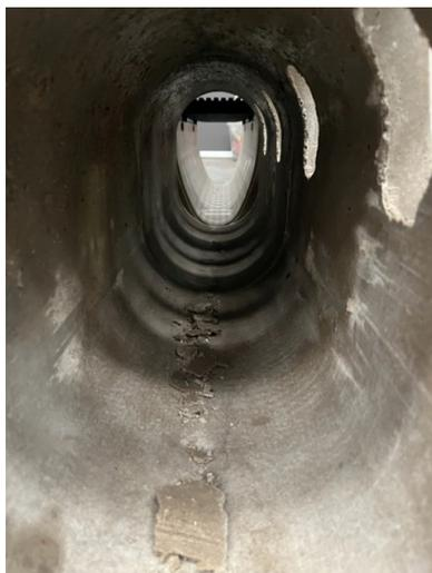
Invert of KerbDrain transitioning into KlassikDrain
